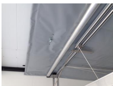
Hook the rod onto the perforated strip and pull the partition wall to the desired position.
