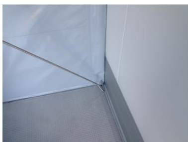
Press the folds of the partition against the wall at the corners to ensure absolute tightness.
